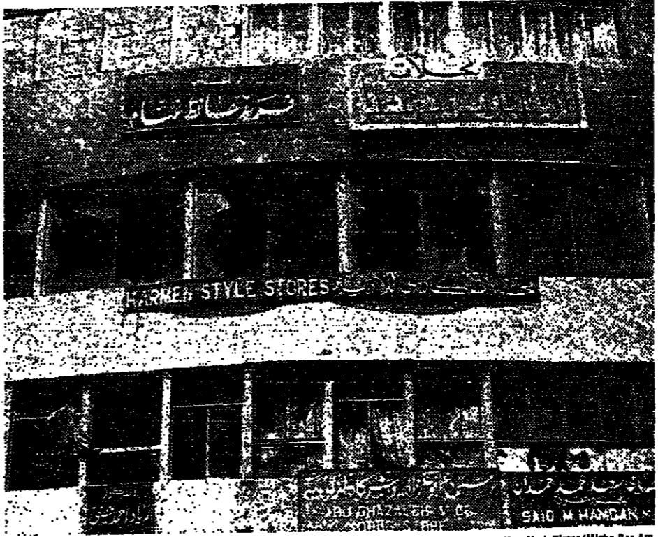
Windows from which Israelis keep watch are shattered from previous outbursts
